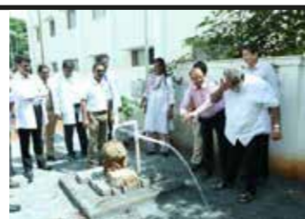
Three borewells dug at Coimbatore Medical College and Hospital (CMCH)
